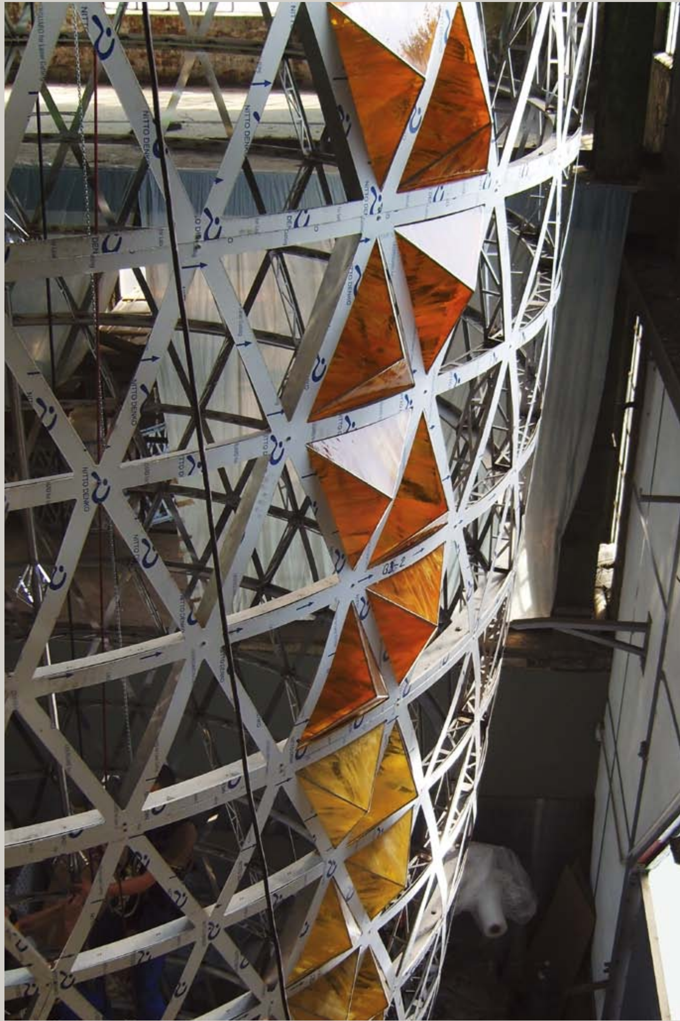
Setting up the Nanuyan Ningbo lighting installation
