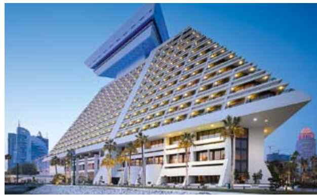
West Bay, Doha, Qatar
